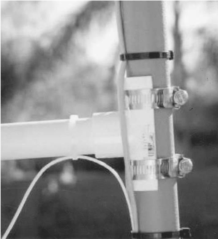
**Figure 7-7** Securing the LSU to the mast.
